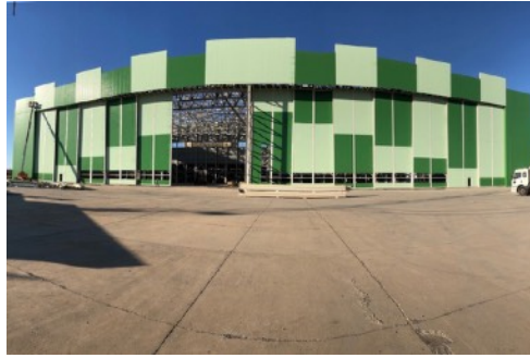
Aircraft Main. Hangar- Bağdat IQ
